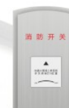
消防开关 Fire-fighting home landing
